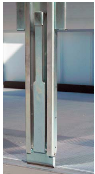
Roof support post
